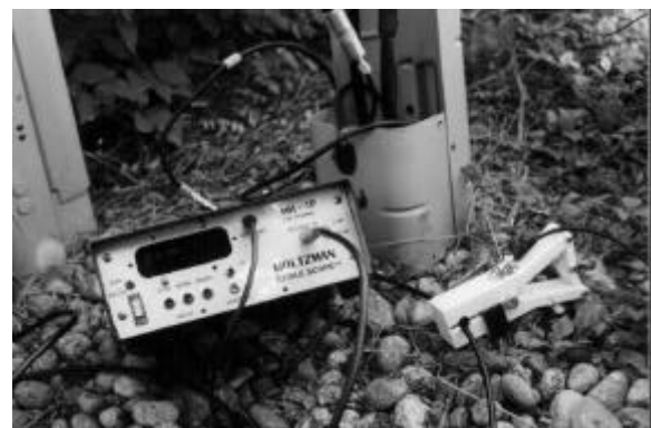
Photo 1. Sheath current induction test at a tap
